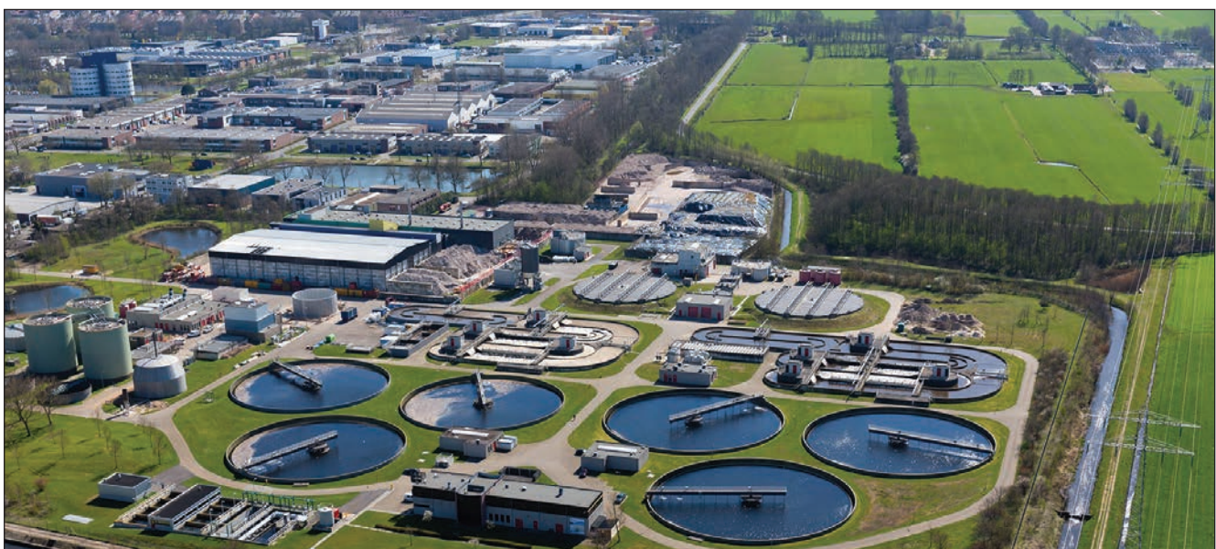
Figure 1: RWZI Amersfoort is one of a total of eight Vallei en Veluwe wastewater treatment plants that also produce electricity and artificial fertilizers as ‘energy factories.’ ©RWZI Amersfoort
